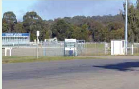
Full perimeter fencing erected around the training facility that is high enough to contain horses.
